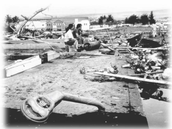
[Parking meters on Kamehameha Ave following the 1960 tsunami. Pacific Tsunami Museum.]
