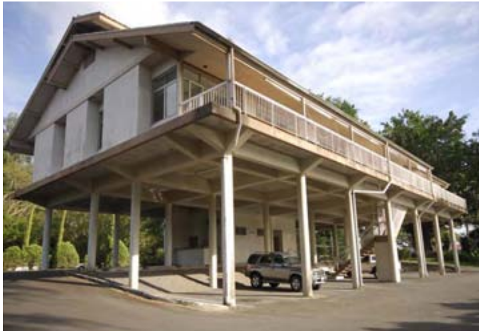
Figure 4-2 – Example of structure in Hilo designed for wave and flood action with modified knee braces on columns.
