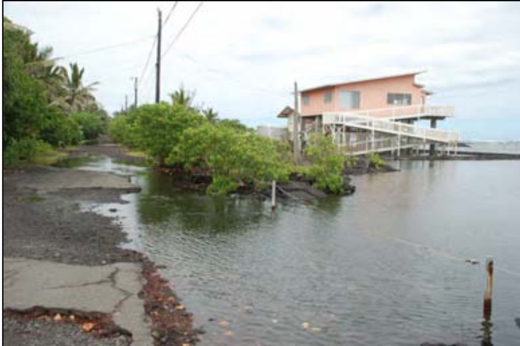
Figure 3-3 - 1:26 PM. – The tide is continuing to rise. Once crossing the road, the water spills over to lower areas mauka of the roadway, and floods properties mauka of the road.
