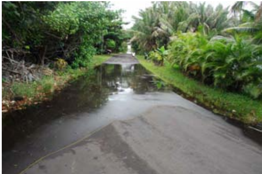
Figure 3-10 – Maximum inundation on July 10, 2006. Although the predicted high tide was less, at 3.13 above MLLW, the inundation is greater. This is attributed to stronger wind and wave setup, but subsidence could have also played a role. Depth of water at the maximum channel depth is 1 \frac{15}{16} of an inch or about 5 cm.
