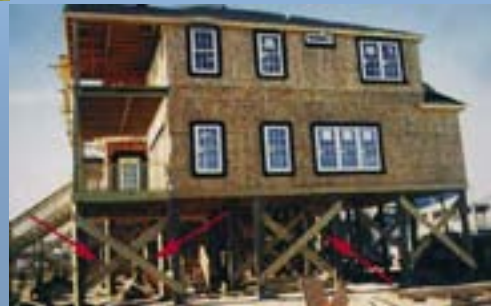
Figure 4-1 – Examples of Coastal Homes with Knee Braces and Cross Braces to strengthen columns or piers that are needed to elevate houses for flood or wave protection (from FEMA CCM).
