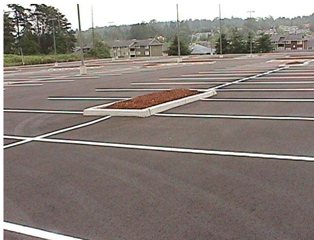
A park-and-ride lot with lighting and pavement.
