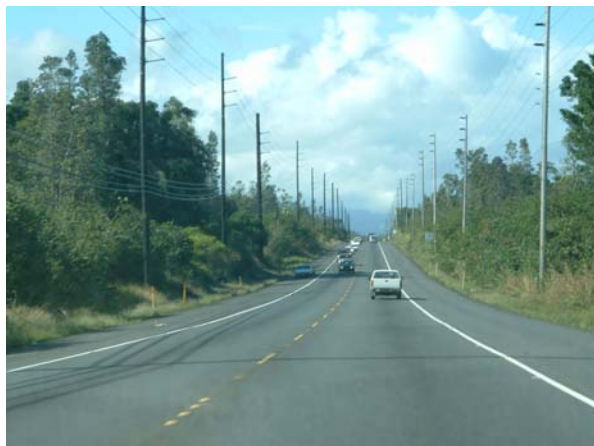
Highway 130, Kea'au-Pahoā Highway
