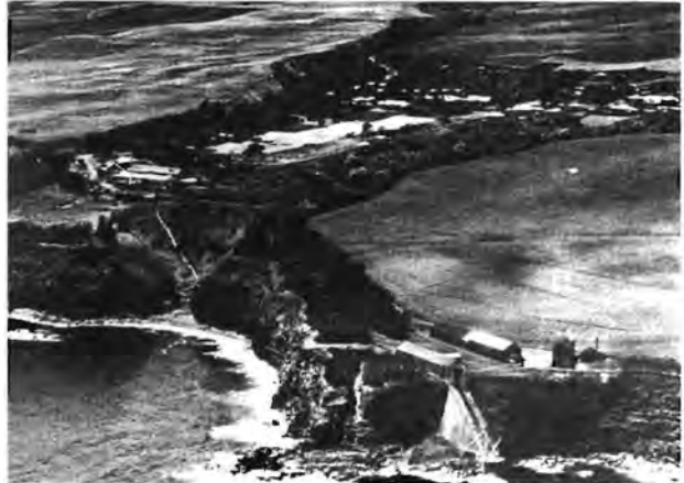
Figure 4. Landing facility at Pā'auhau ca 1920. Note the substantial masonry ramp supporting a steep incline cable railway, and the wharf and derrick at seaside. Pā'auhau Mill and village were situated between two major gulches of Mauna Kea. That is cane field 001 adjacent to the cliff-side warehouses. Pā'auhau Sugar Company.
