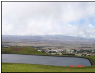
One of the reservoirs that services the Waimea Water Delivery System
